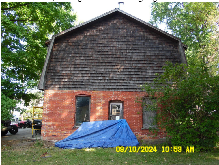
Looking northwest at south side of garage
