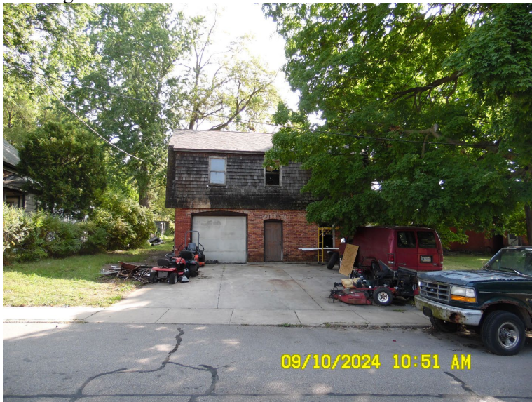
From 5 th Street, looking northeast at the garage
