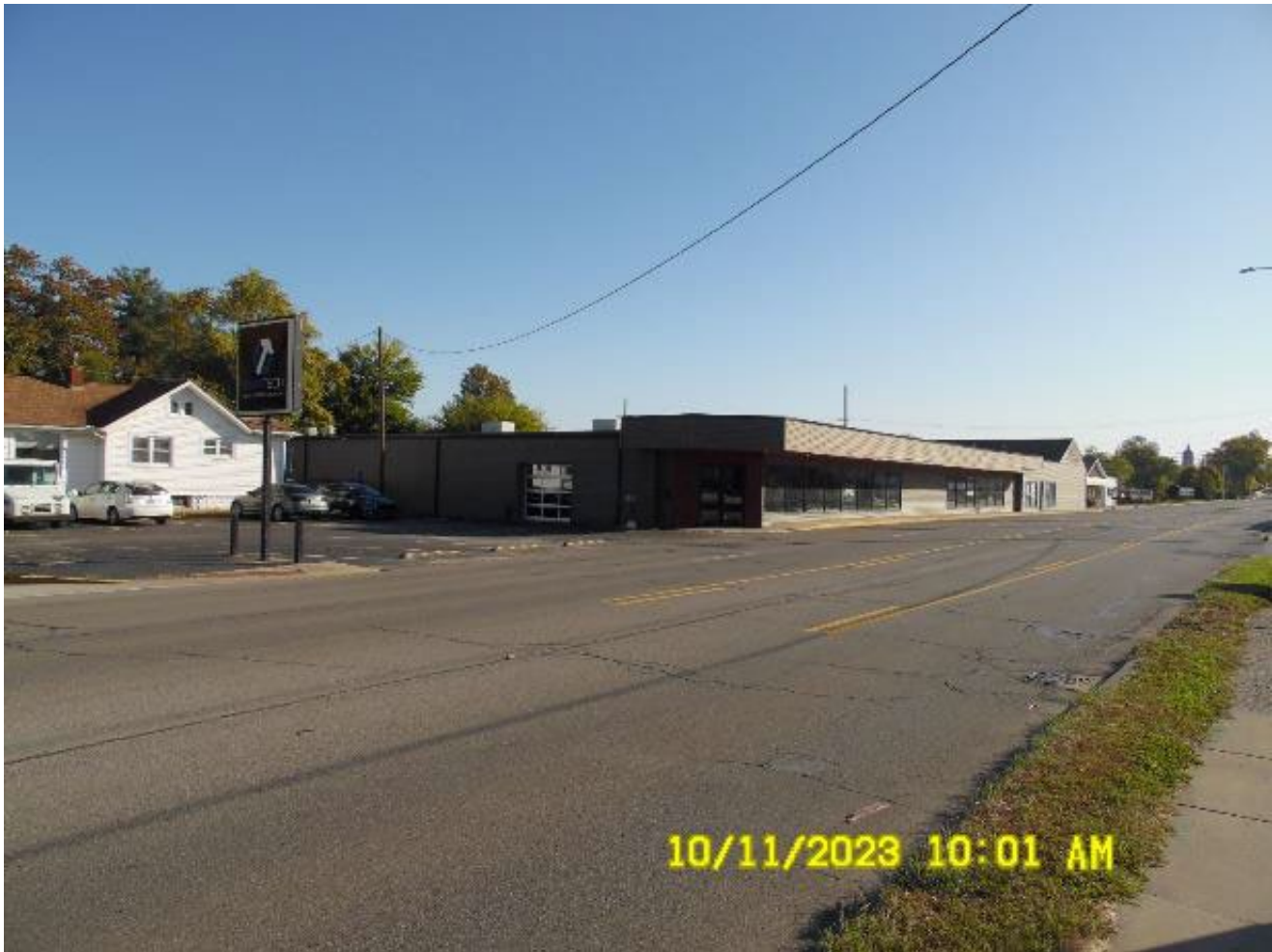
Looking northeast across Lincoln Avenue
