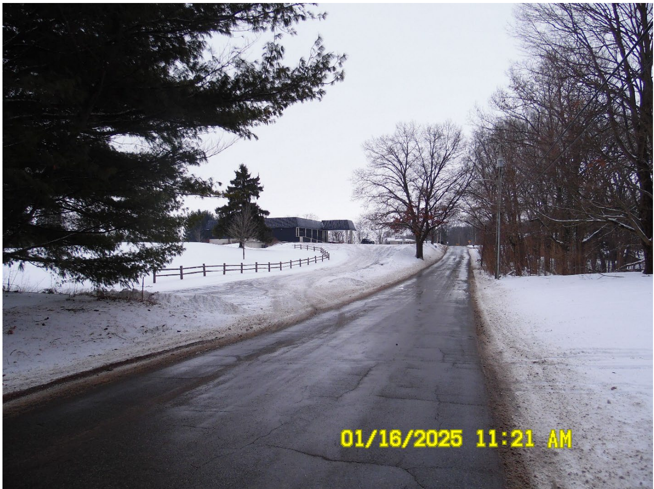
Looking east along Hackett Road
