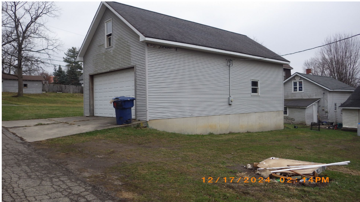
Figure 2. Looking southeast at detached rear garage and rear entrance of 211 Queen Street.
