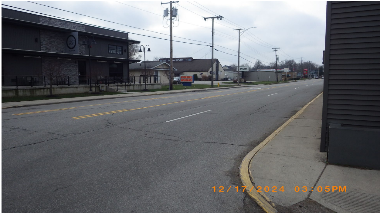
Figure 4. Looking east from Denver Street. The front of vehicle would be encroaching in the westbound lane to achieve adequate sight distance.
