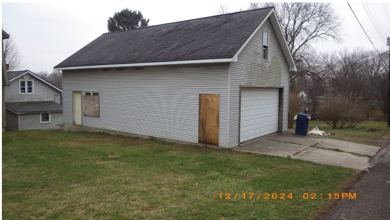
Figure 3. Looking southwest at detached rear garage and back of 211 Queen Street.
