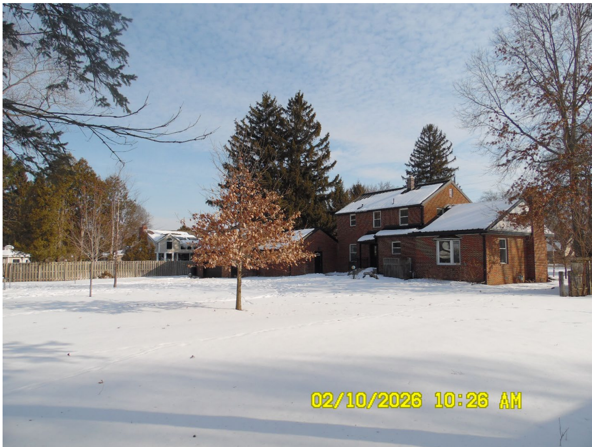
Looking northeast at rear of home
