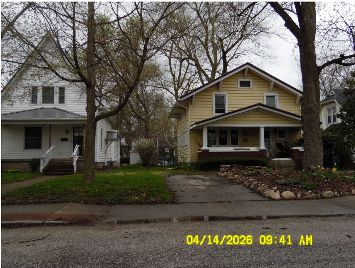
From 8 th street looking west along the south property line
