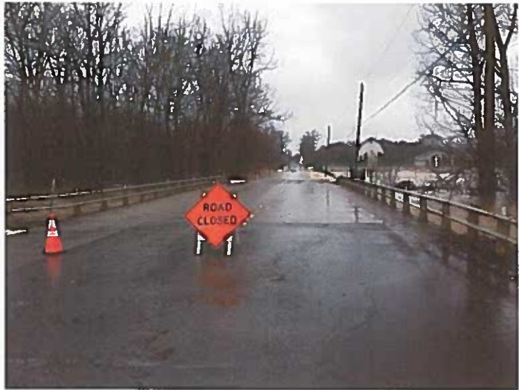
Figure 41 Flooded Roads and Street Closures
