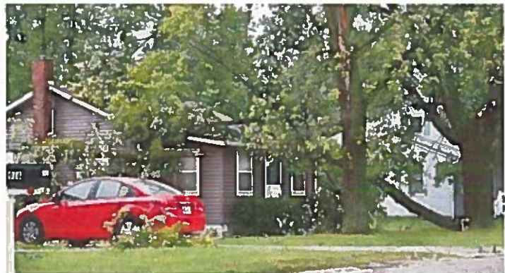
Figure 43: Damage from a Windstorm
