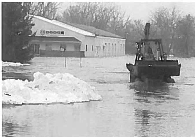
Figure 52 Flooding caused by Snow Melt
