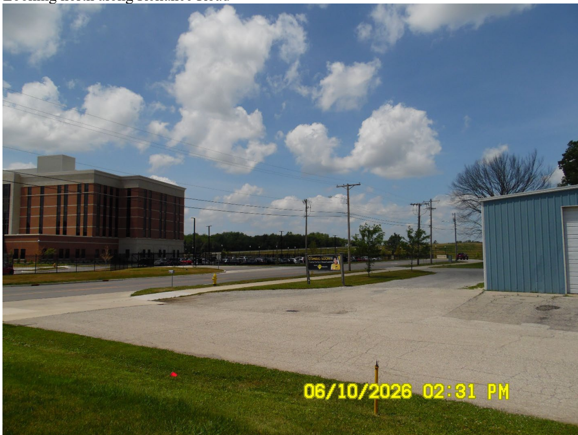
Looking northwest across Reliance Road
