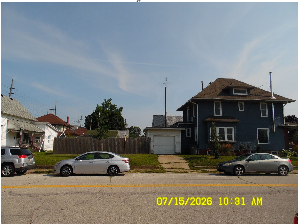
From Clinton Street looking north
