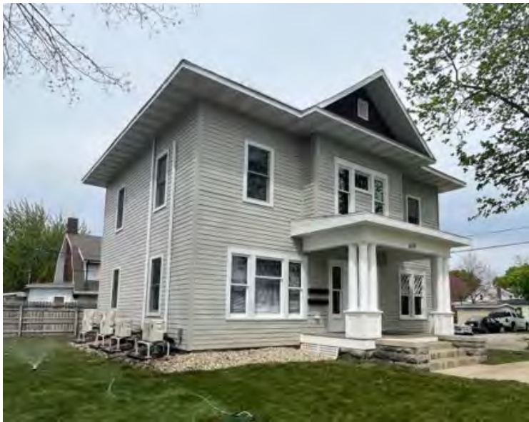
409 E Madison St. Multi Family Rehab project added 4 new affordable rental units
