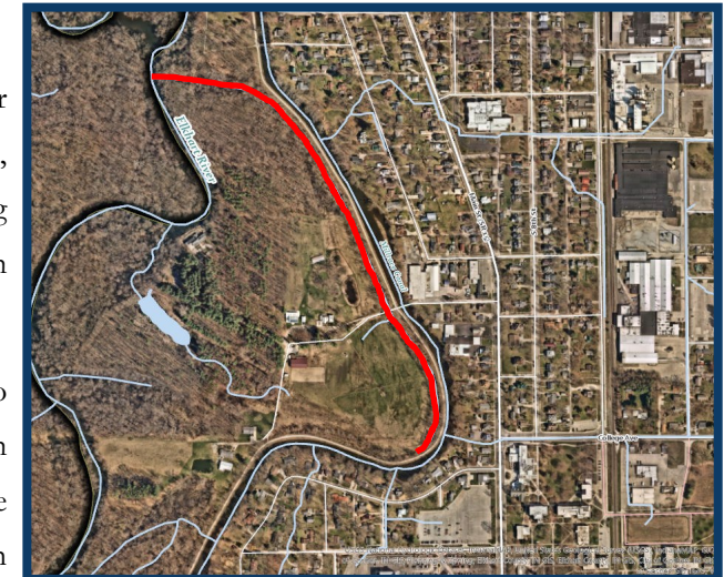
Wellington Ditch highlighted in red.
