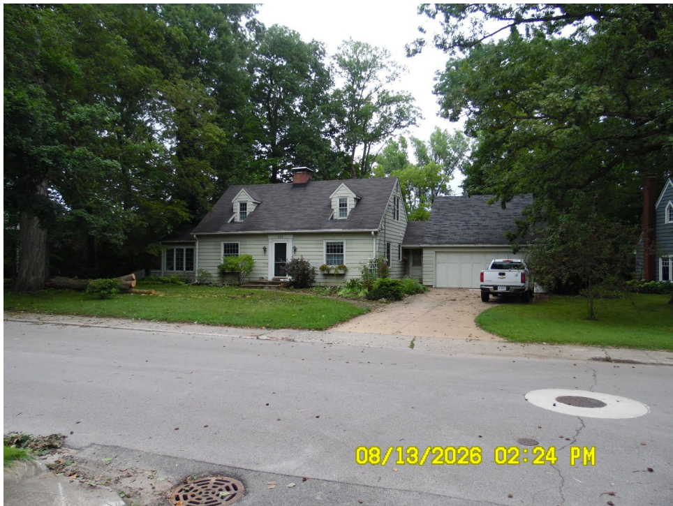
Looking north across Gra Roy Drive at the front of the home
