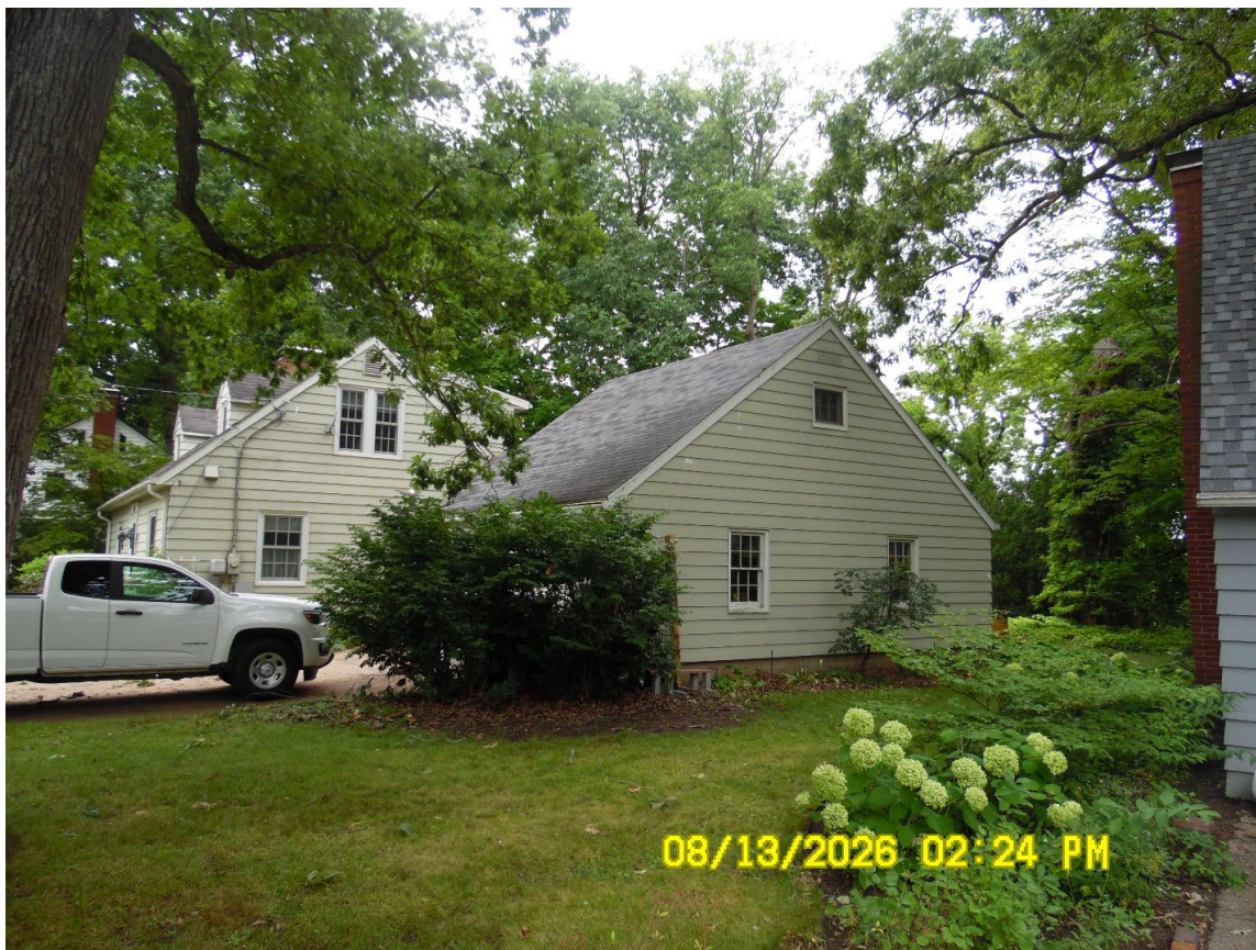
Looking west at garage in question
