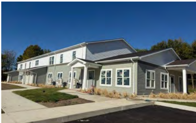
This building is 11 units for those who are aging out of foster care.
