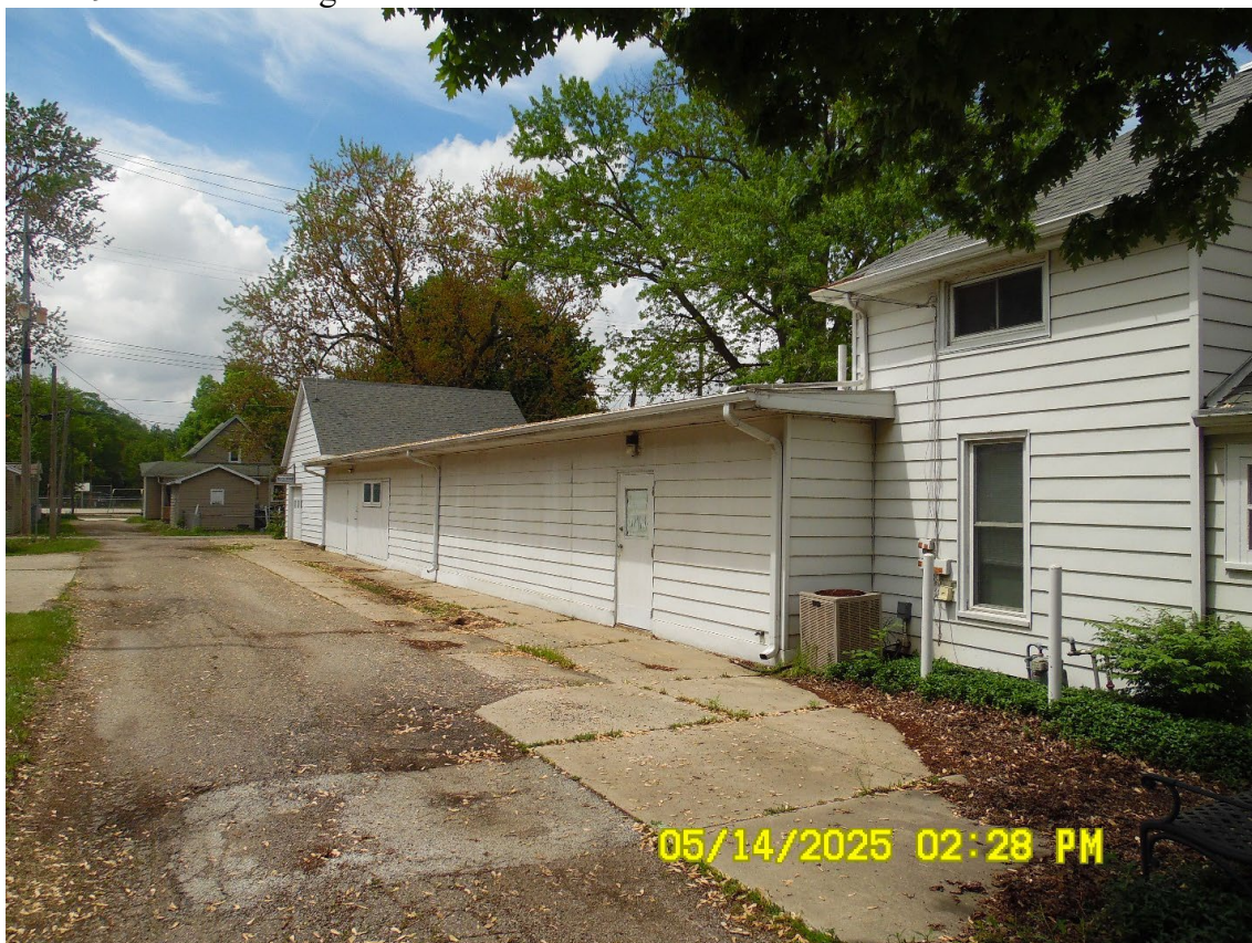
From alley looking west along south side of building
